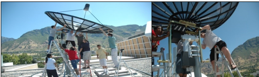
Figure 3-9: Mounting the 4-meter dish upon its azimuth/elevations motor/gearbox assembly.
