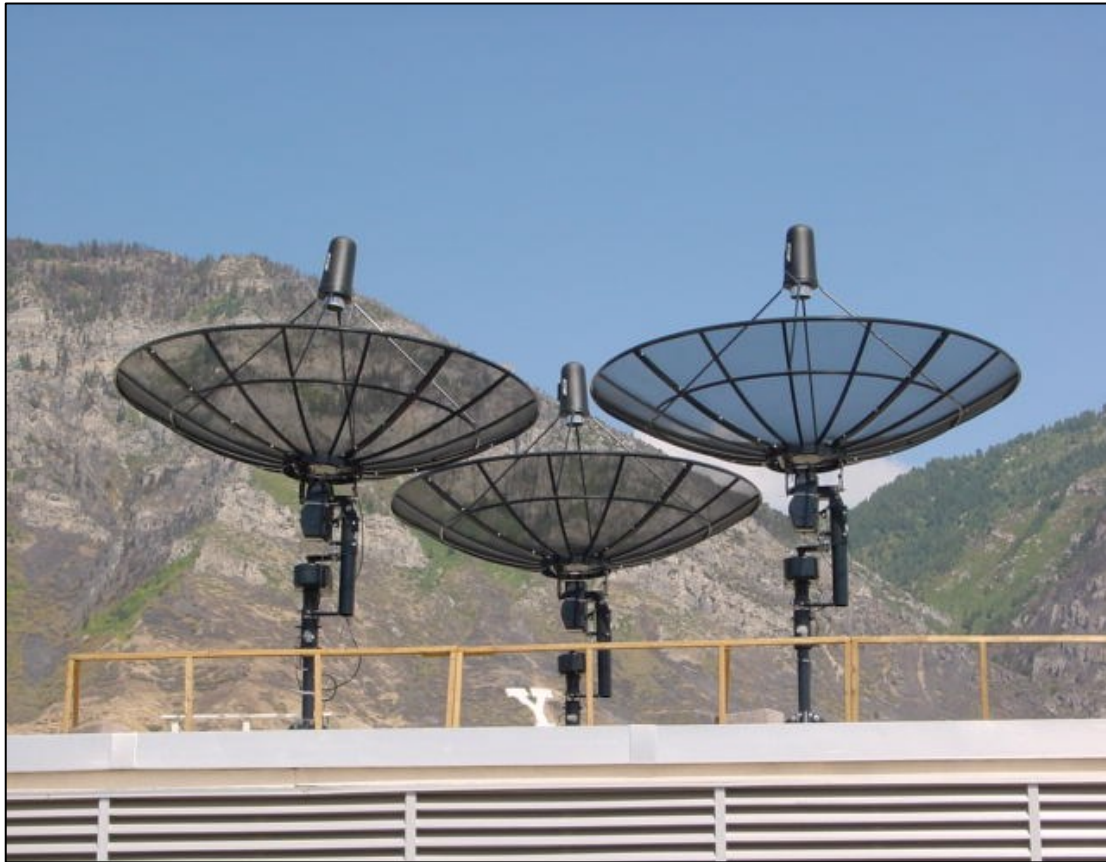
Figure 1-7. VSA Located on Clyde Building. Three of the Six Array Antennas are shown here. Photo courtesy the BYU Electrical Engineering Research Group of Dr. Brian Jeffs and Dr. Karl Warnick.
