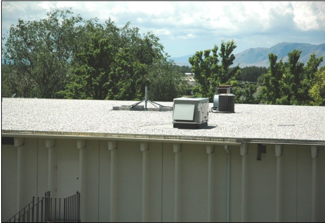
Figure 5-4: The old KBYU building site, showing the antenna mounting base on the roof in the center of the photo. Photo, courtesy of Scott Daniel.
